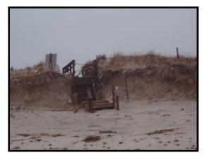
This is the second set of stairs – most easterly set. Bottom part is concrete which remained but the rest of the stairs are gone.
