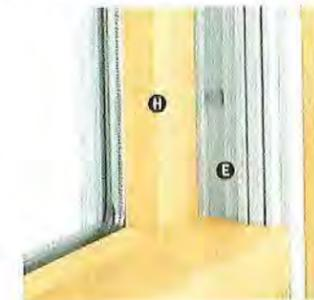
**F** Weatherstripping throughout the unit provides a long-lasting, energy-efficient, weather-resistant seal. For the top and bottom rails, an encased foam material is used. The head jamb liner and sill have a rigid vinyl rib that the weatherstripping material compresses against. At the check rail, compressible vinyl bulb material is used. Side jamb liners use leaf-type weatherstripping with foam inserts.
