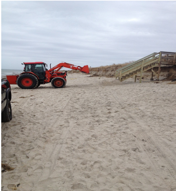
A backhoe makes some minor adjustments to sand during step rebuilding.
