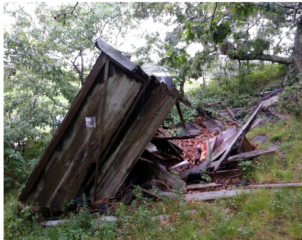
Winders cottage prior to demo and debris removal.
