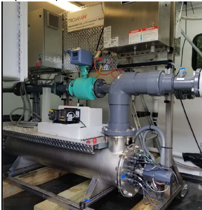
Figure 2.13: Trojan Pilot UV System Photo
