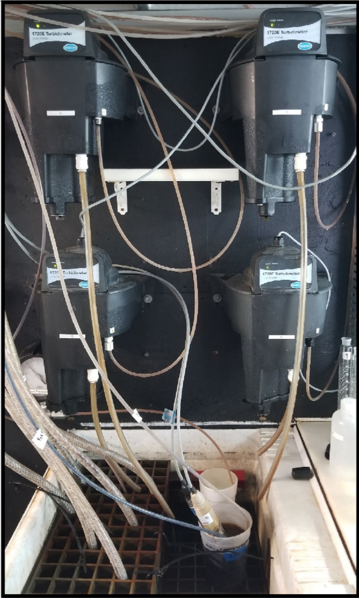
Figure 2.07: Sample Sink and Hach 1720E low range turbidimeters
