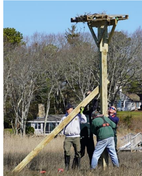
Osprey Pole construction, Centerville River.
