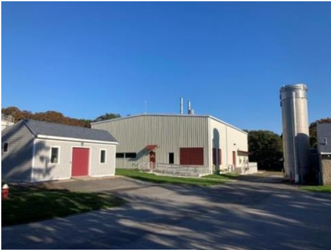
Harold E. Tobey Maher Water Filtration Plant
