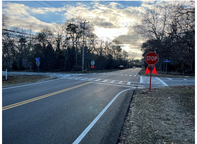
Crosswalk and Stop Bar Installation
