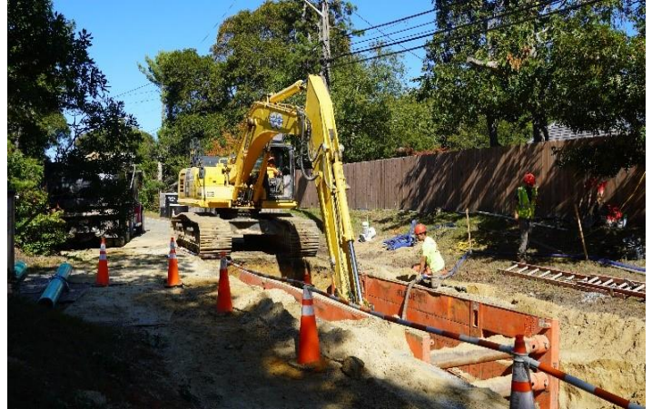
Strawberry Hill Road Sewer Expansion Project
