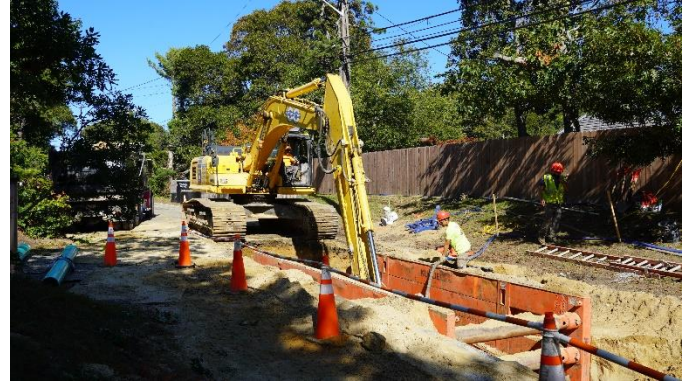
Strawberry Hill Road Sewer Construction
