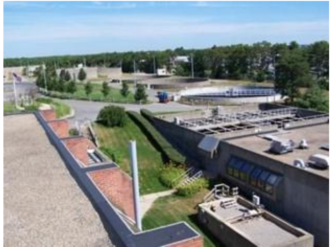
Water Pollution Control Facility - Grounds
