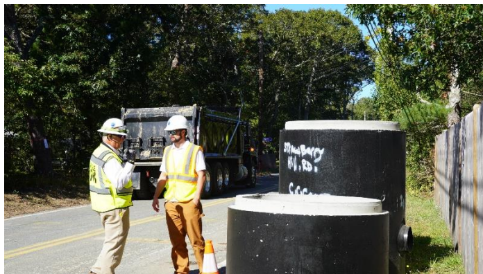
Sewer construction on Strawberry Hill Road
