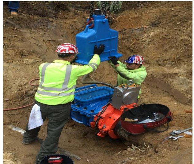
Pipe Replacement Project -2023
