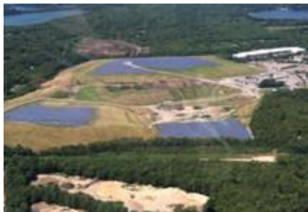
Solid Waste Facility – Aerial View
